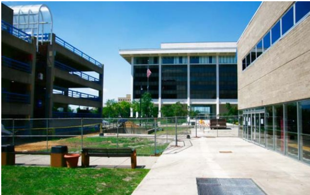
The PCCC entranceway as it looks today. PHOTO BY PATRICK YEAGLE
